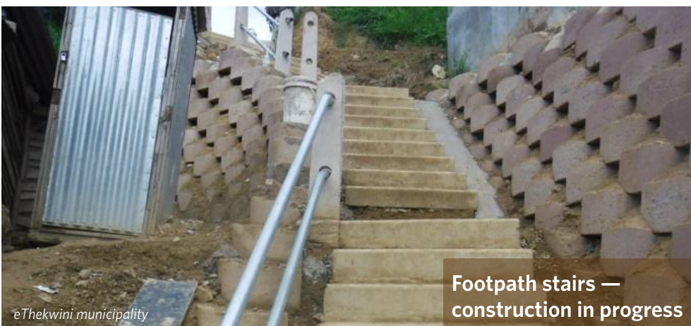
Foot path access — construction in progress
